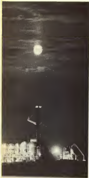
Desalination plant at Mangyshlak Peninsula on the Caspian Sea
